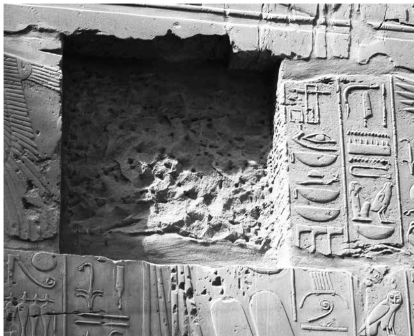
Figure 8. Missing patch block on north wall; detail of plate 179
