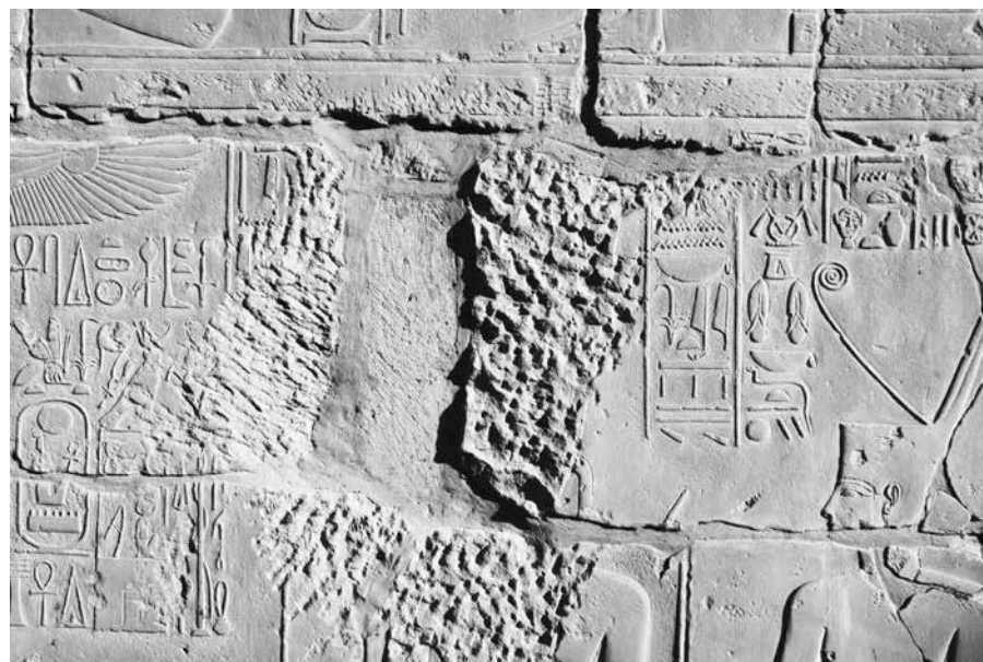
Figure 2. Quarry damage; detail of plate 209
