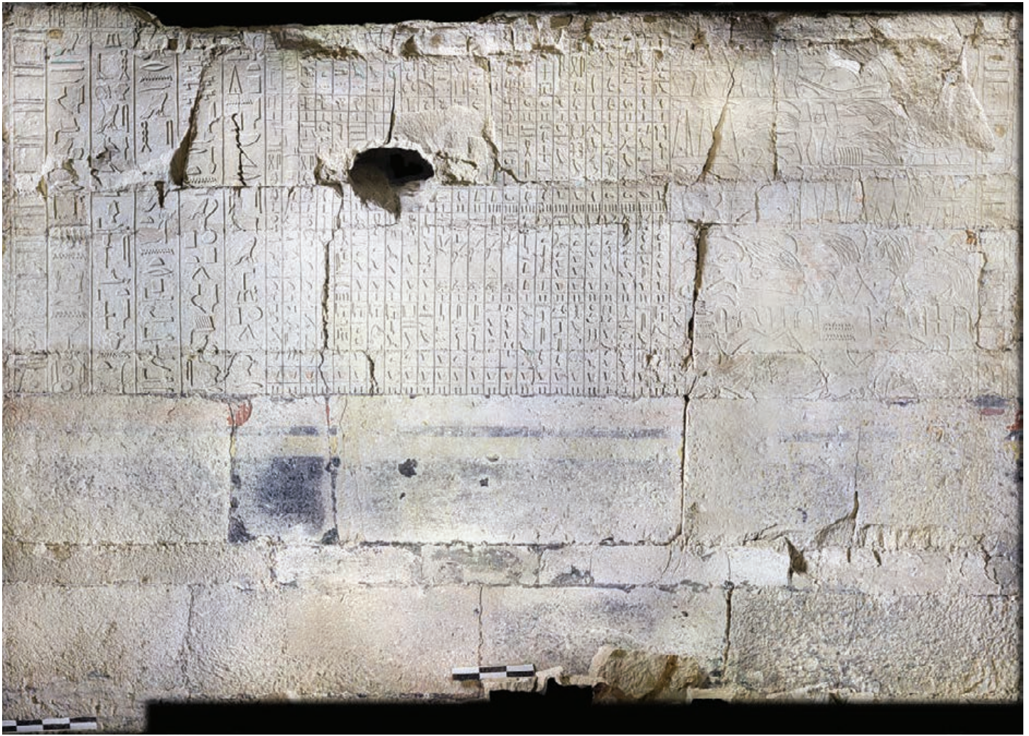
Figure 6. East wall of the southern (main) burial chamber of Khentika, showing damaged areas. Photo by Dr. Osama Bassiouny.
