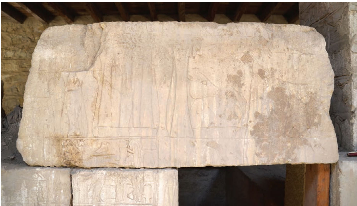
Figure 5. Detail of the south wall of Room IX, showing water damage from rain. Photo by Anna-Latifa Mourad-Cizek.
