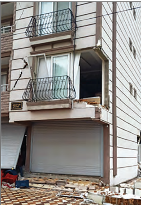
Figures 4–5. The excavation house after the earthquake of February 20.
