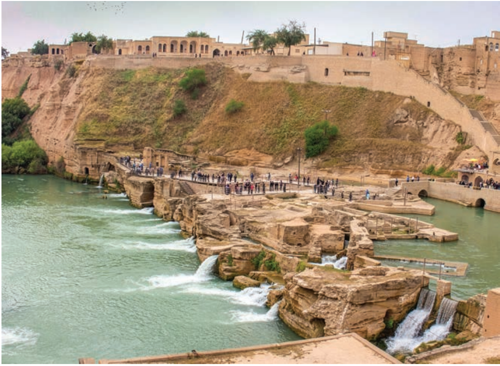
Figure 5.3. An enormous Sasanian-Persian water system at Shūshtar. Photo by Razie Amirian, Wikimedia Commons.
