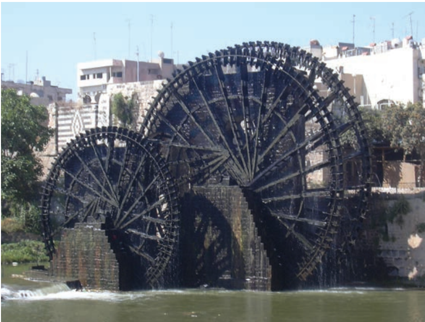
Figure 5.2. Noria water-lifting wheels, originally constructed in early Islamic times. Hama on the Orontes River, Syria. Photo by H. Frank, Wikimedia Commons.
