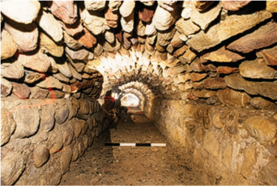
Figure 5.22. Roughly corbeled vault of underground channel leading north. Photo by T. Springett.
