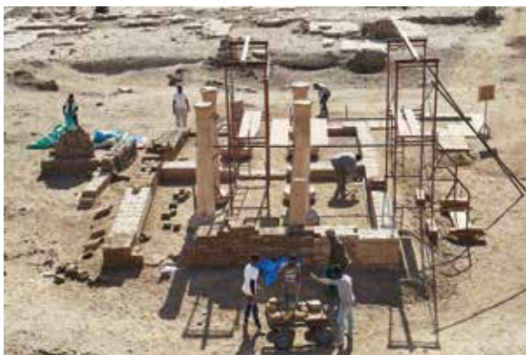
ABOVE: Frank, Saber, and Johannes laying stone slabs (February 27, 2018). Photo by Ray Johnson.
